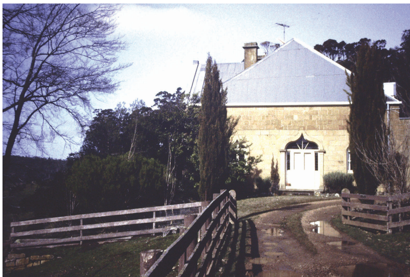
Fig. 2. Fonthill House, entrance front. The paler stonework was sheltered by an added verandah for almost a century. © Author.
